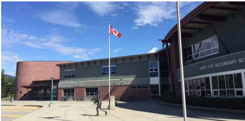
Terry Fox Secondary School in Port Coquitlam. Photo courtesy of SD43.
